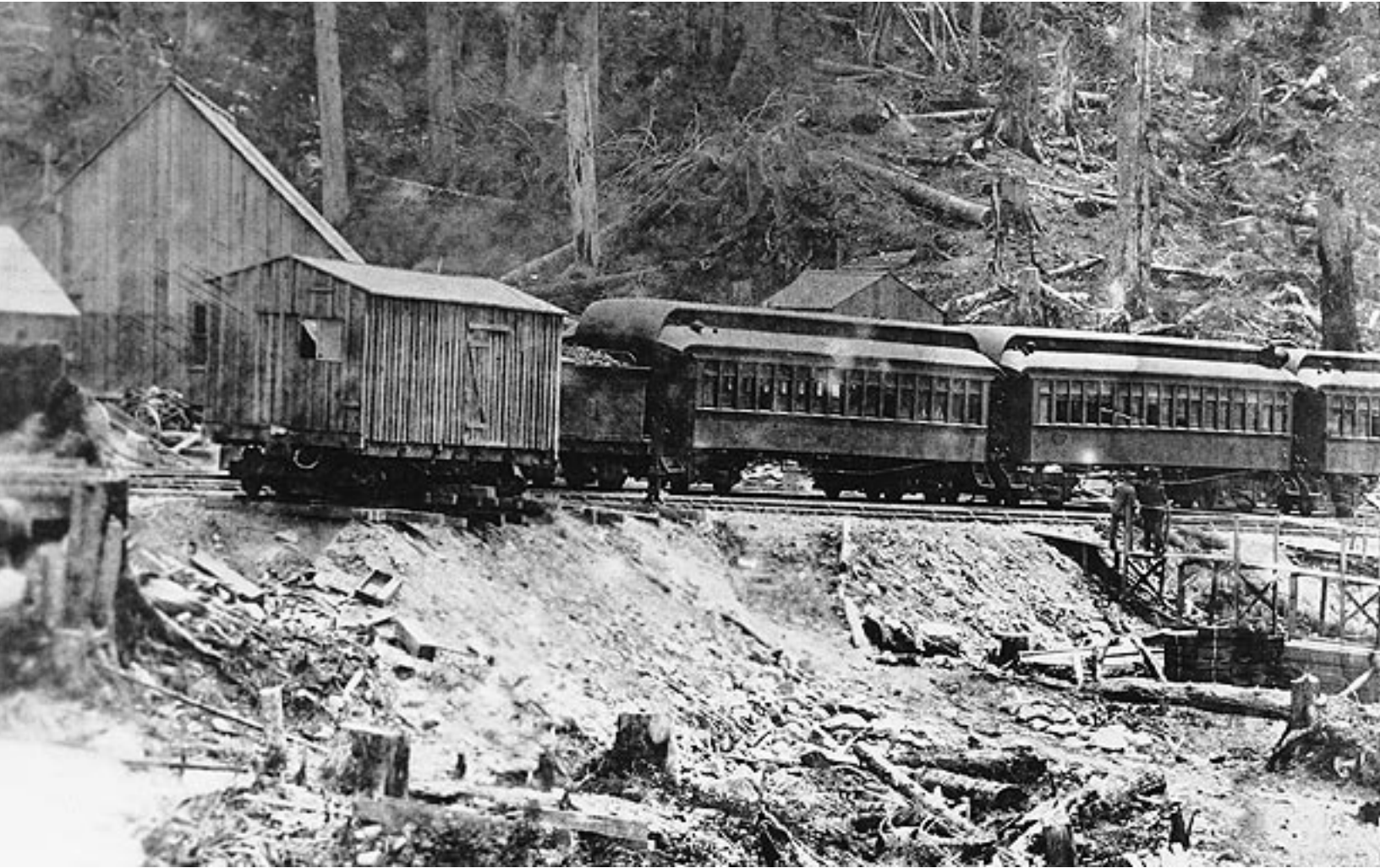
A small portion of an 1894 photo of Monte Cristo. The original negative is 18 inches high by 36 inches wide. Locomotive #3 of the Everett and Monte Cristo Railway hides behind a crummy (work car) while waiting to pull the daily passenger train to Everett. The building behind the crummy is the railway station, which was originally a sawmill erected by the mining companies to supply timber to their mines. ( Frank LaRoche photo )
